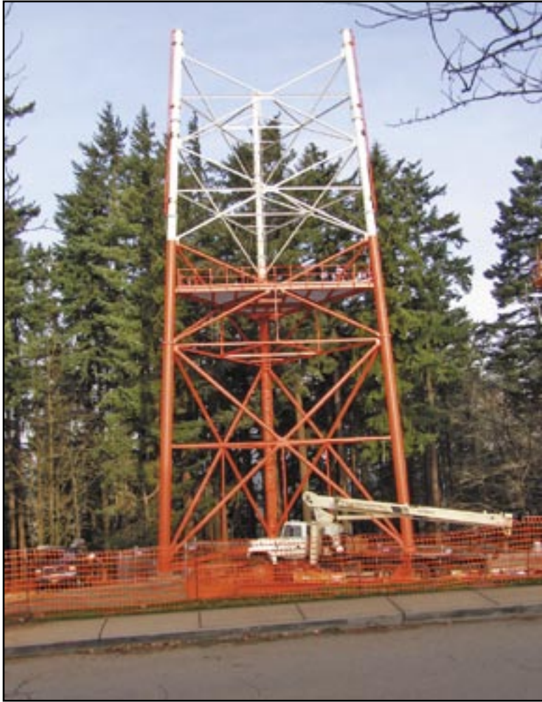
The new Council Crest tower on February 19, at about 100 feet.
